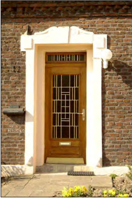
Türe in Haverslohe
